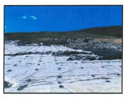
challenging to completely cover at the end of the day. The access roads are in very good, maintained condition. Specifically, waste was being pushed into the working face with a CAT D6 dozer and compacted with a CAT 836K waste compactor. Daily cover soil was being placed with a D6 CAT dozer. Daily cover soil was being hauled and dumped with a CAT 745 end dump truck. The number and size of the operating equipment are consistent with waste industry standards for this size of a facility.
